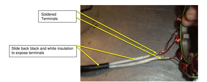
Figure 3 - Terminal exposure
